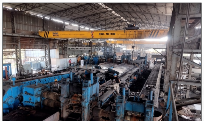
Structure rolling mill
